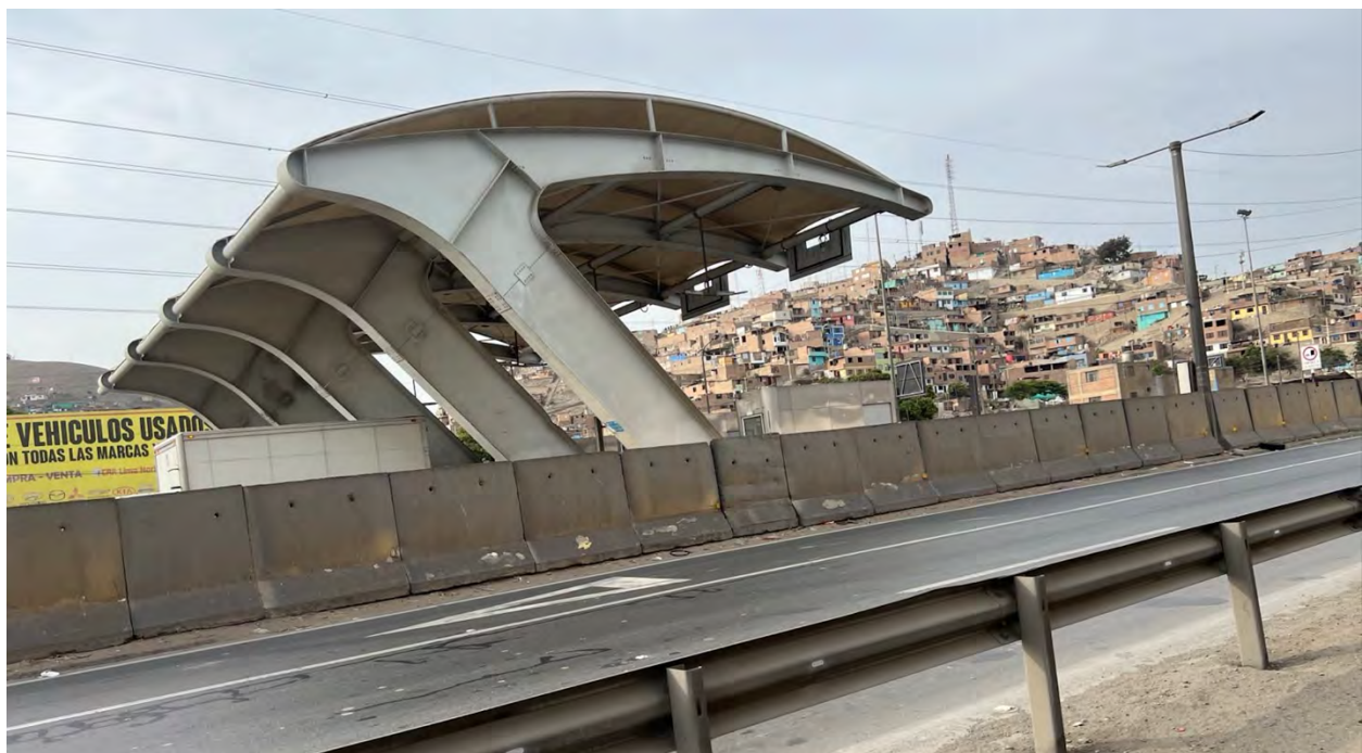
Brookfield's Rutas de Lima toll plaza, Chillón, appears to swallow the Quechua-speaking shantytown trapped behind it.
